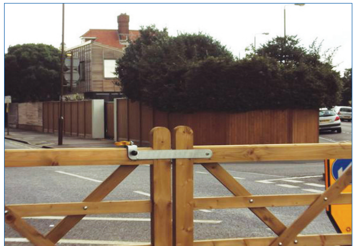
Detail of the gates 'loop over' fittings
